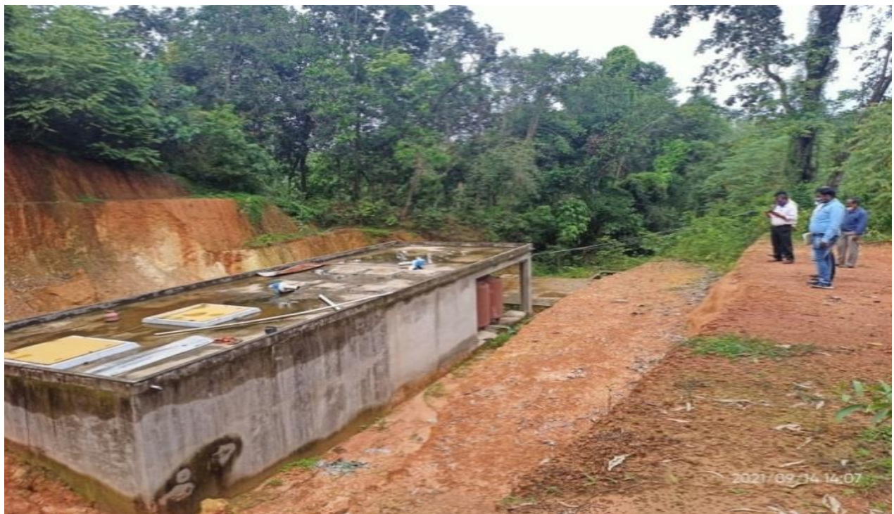
Provision of Sewage Plant at Vivekananda College, Puttur
