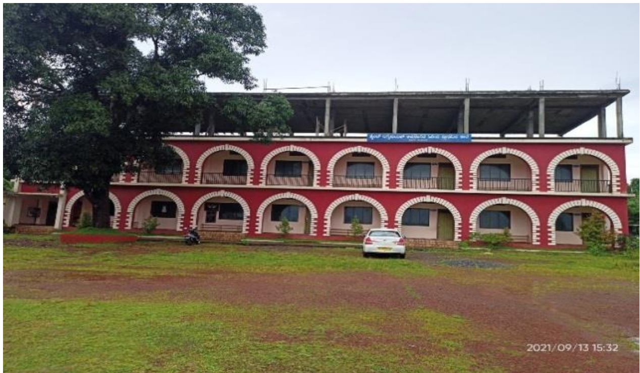
Provision of School building
