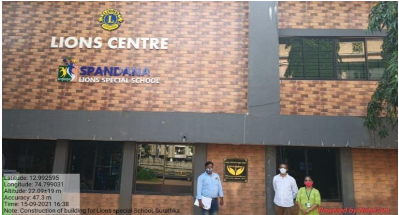
Provision of school building
