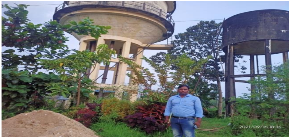
Bajpe Village Water overhead tank
