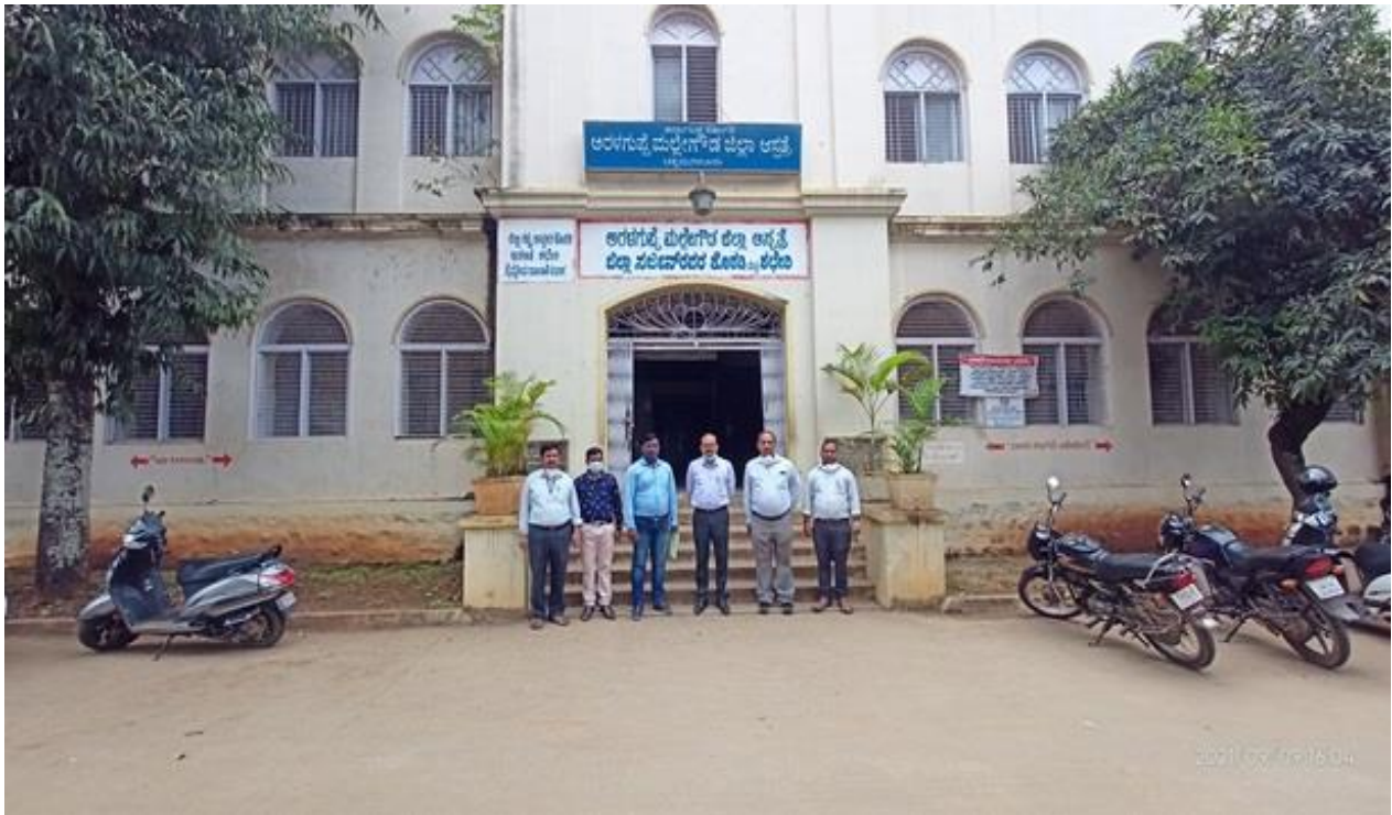
Entrance of the Hospital
