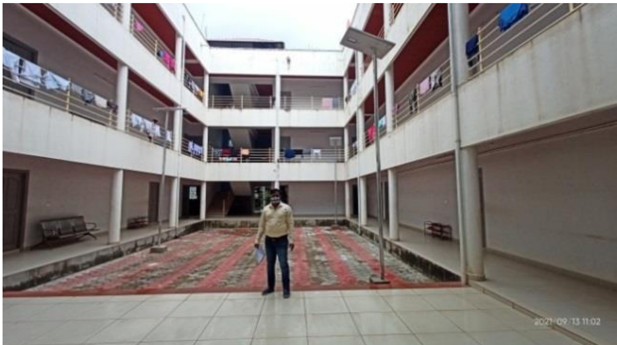
Provision of solar light
